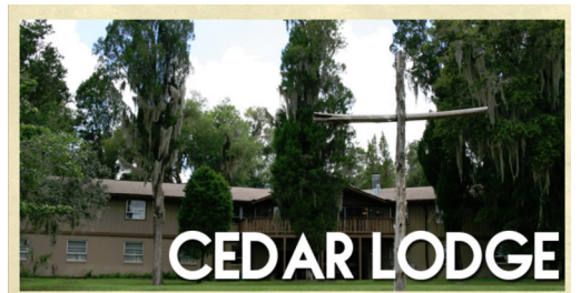
This central lodge at Cedarkirk is the location of the main offices, 2 dining rooms/meeting rooms, upper and lower back porches, and a library. In addition, there are three wings of housing accommodations including both family-style and dormitory-style rooms.
